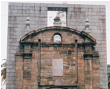
The door of the Ciudadela is the entrance to the colonial city.
